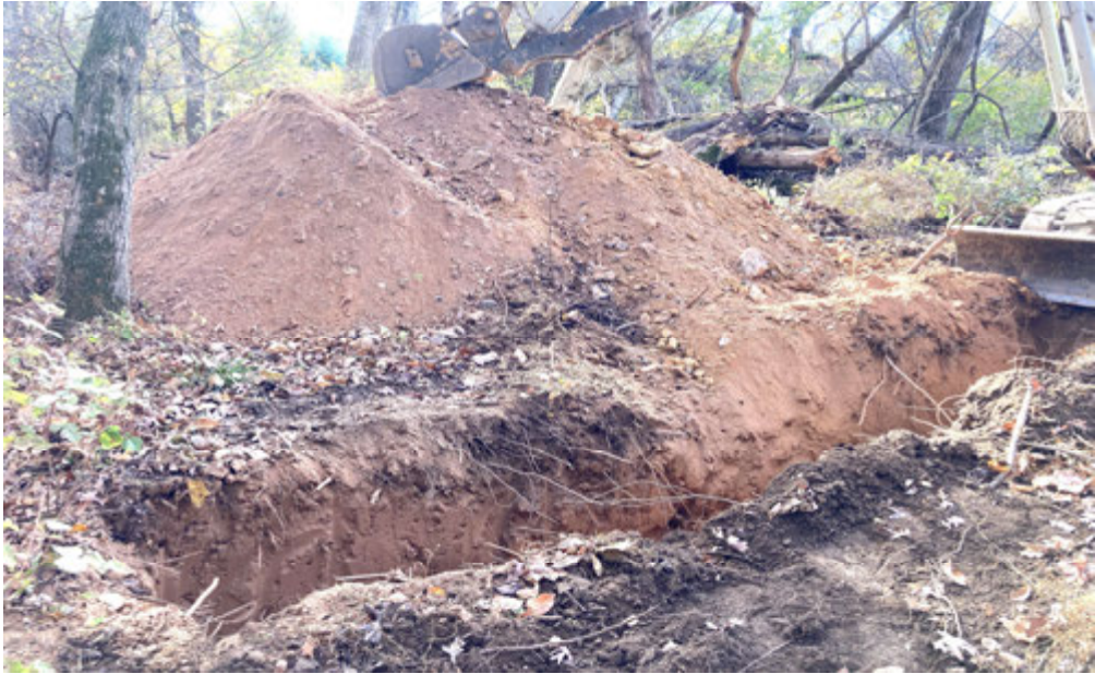
Typical excavation for “perc” testing.
